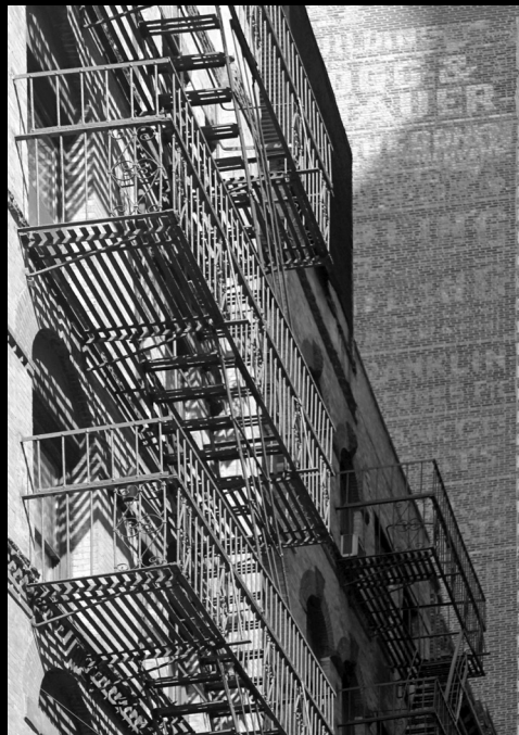
Fire Escape 1509 Fire Escape 1304 V Fire Escape 151
